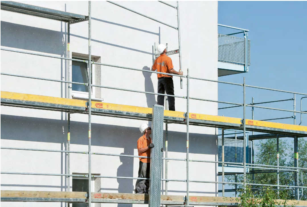
The “mounted-ahead guardrail” – for instance, on PERI UP Easy facade scaffolding – secures the next level before the scaffolder steps onto it.
